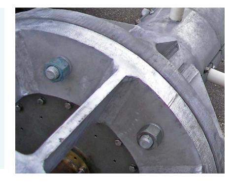
There is enough vertical room in this wedding cake to clear a 3-1/8" EIA transmission line and elbow. There are several designs that could have been used. The wedding cake could be part of the bottom antenna pylon, be a separate section or be integrated into the top antenna pylon. All three methods have excellent mechanical strength.
