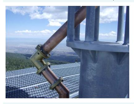
The picture to the left shows a close up of a wedding cake that is part of a bury section. The antenna is mounted on top the wedding cake and is bolted in place. The transmission line comes in at a 45 degree angle and attaches to an EIA flange on the bottom of the antenna.
